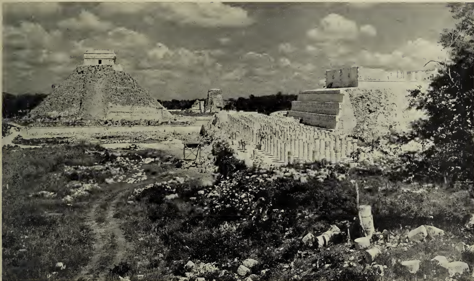
LOOKING WEST ALONG NORTH COLONNADE TOWARD TEMPLE OF THE TIGERS At left center is base of back wall of West Colonnade and beyond it the Castillo. At right appears Temple of the Warriors, showing unrepaired east face of pyramid. South side presented same appearance before excavation.
